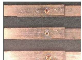
Welding of bus bars
